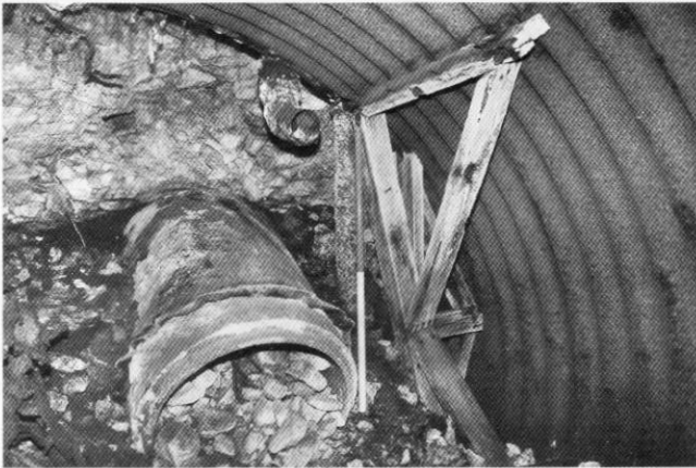
Arundel OB: internal dividing wall with door frame still in place
